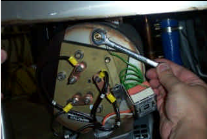
Removing the imperial brass fitting.
